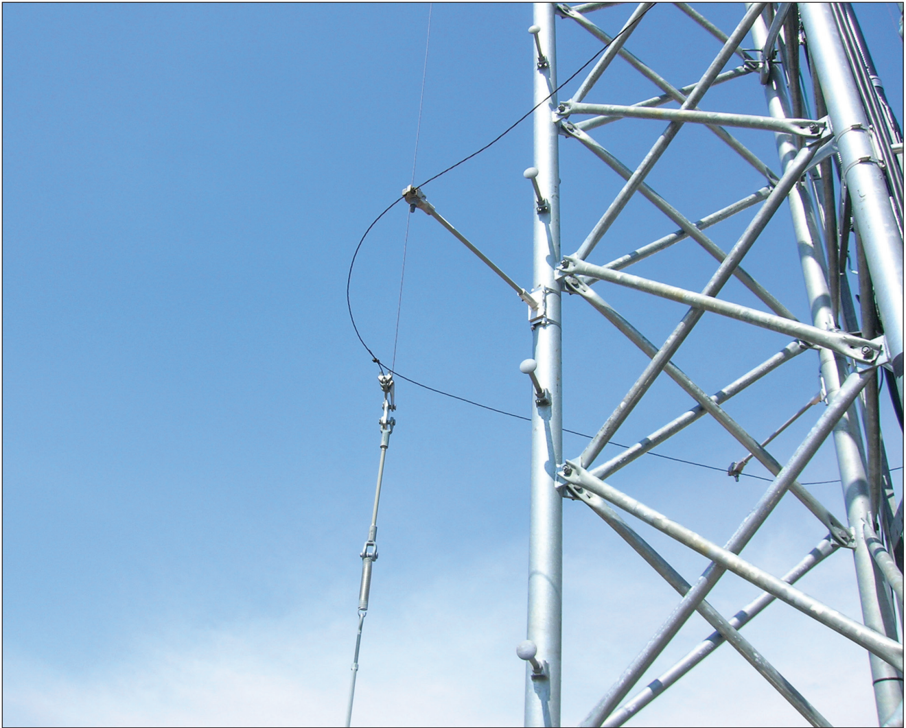
Stand-off insulators support a portion of the wire skirt engineered specifically for the cellular tower. Photo courtesy of Waterford Consultants/Larry Giessman
